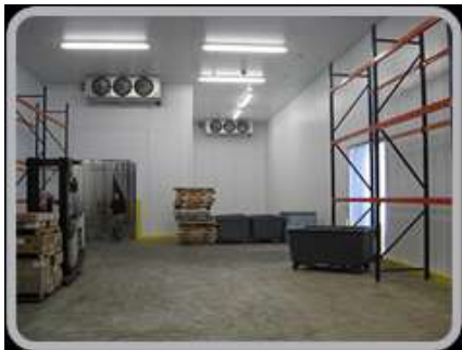
Cold Storage work
